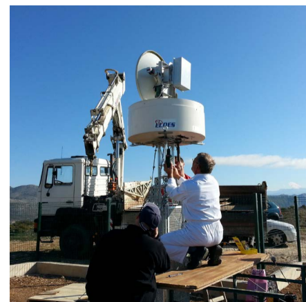
The works on the radar installation
